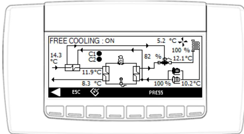
Fig. 47 Water/water units - Specific Master freecooling screen showing readings and devices
