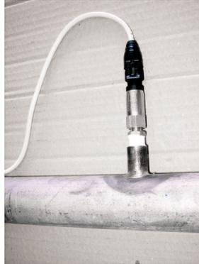
*Fig. 17 Connection of a pressure sensor*
