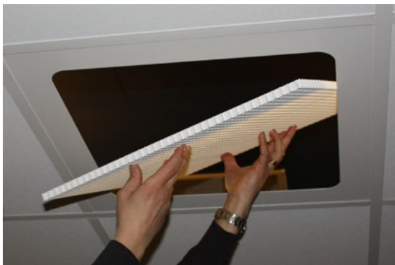
Figure 2. Raster installation in ADAPTER.
