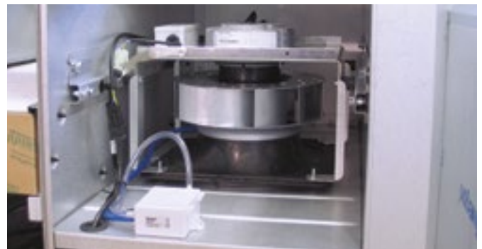
Direct-driven fans with EC motors.
