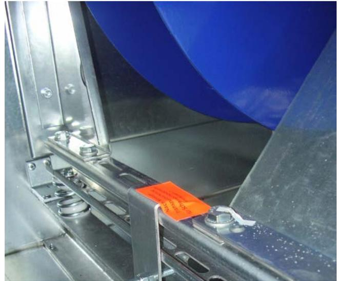
After completion, a test run is to be carried out to check performance and direction of motor rotation.
