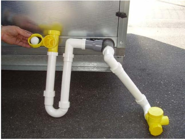
The siphon height should be accurately determined, dependent upon the pressure head.
