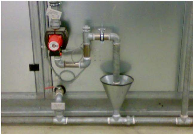
Horizontal drainage pipes must have a sufficient diameter and slope gradient, as well as ventilation and bleed properties for fault-free water drainage.
